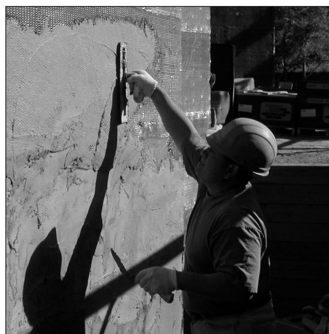
Figure 1B - Applying Scratch Coat of Mortar
