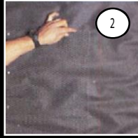
Install corrosion-resistant metal lath.
